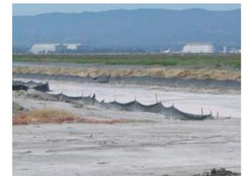
View of NASA Ames Research Center, Moffett Field from Cargill Salt plant in Newark, CA. The excavation work in the foreground shows construction of graded crystallizing ponds. The bottoms of the ponds are made of naturally occurring clay.
